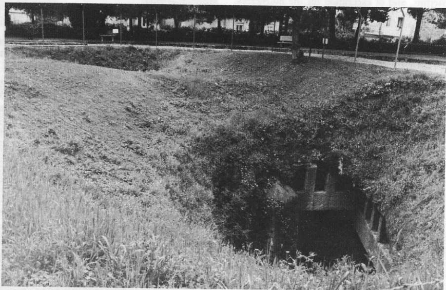
The two places where the tunnel roof was penetrated by the German explosions have been grassed over and retained.
